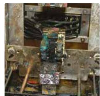
*The effects of corrosion (top) on a circuit breaker, 26 months after moisture contamination and (bottom) on relay contacts. Damage is clearly leading to failure.*
