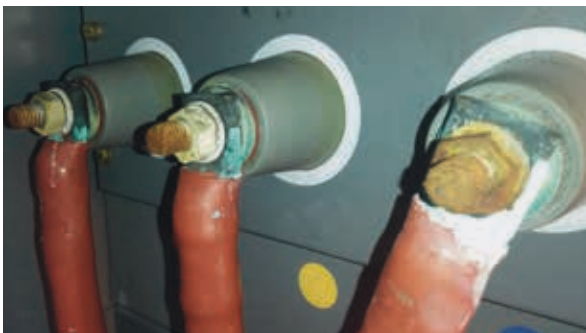
Evidence of PD at site brought to light by UltraTEV Survey
